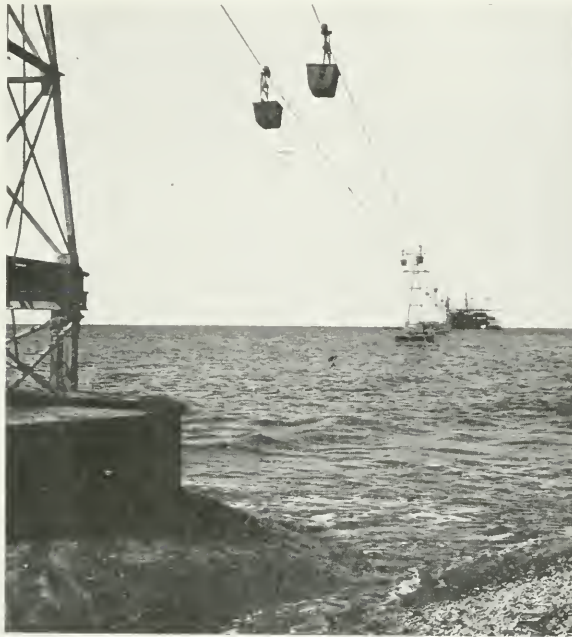
Marine Terminal at Thio.
